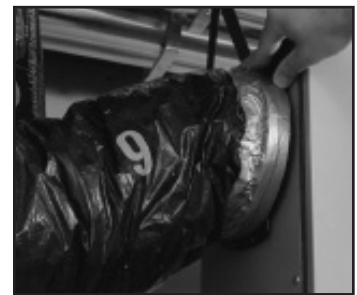
figure 7.4 Slide collar on the unit.
