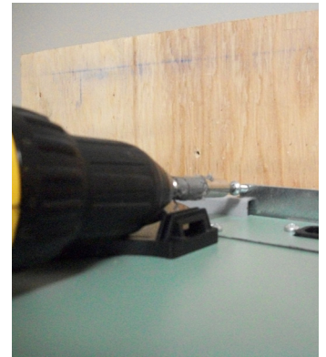
figure 6.4 Proceed to secure HRV to bracket with the two #8 x 3/8" screws.
