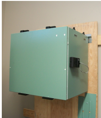
figure 6.2 Hang HRV to wall mounting bracket.
