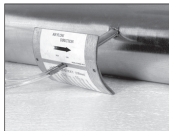
Inserting Air flow grid in duct
