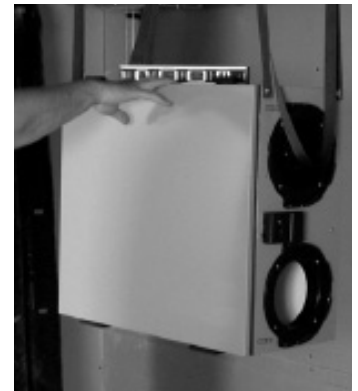
figure 6.7 When completing the procedure make sure that the HRV is leveled.
