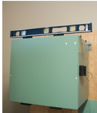
figure 6.3 When completing the procedure make sure that the HRV is leveled.
