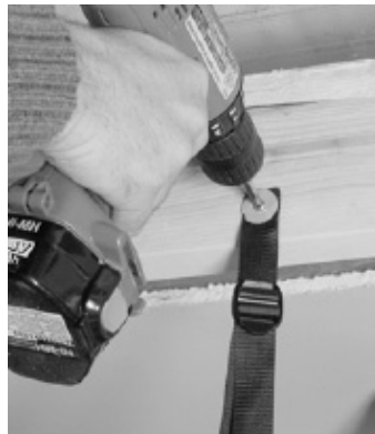
figure 6.5 Attach your four straps to the floor joist making sure that you attach thru the washers and the grommets.
