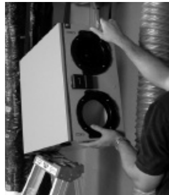
figure 6.6 Pull on the middle strap and gently push upward on the unit. Then repeat procedure on other side.
