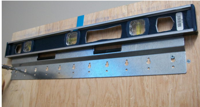
figure 6.1 Installation of the wall bracket. Secure with two #10 x 1 1/4" screws.
